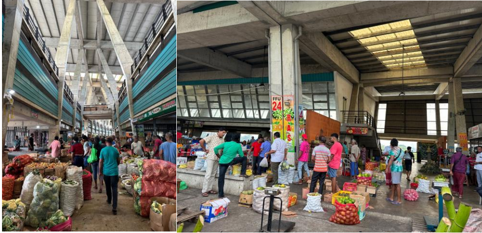
Figure 1: Excessively utilized ground floors and abandoned upper floors at Manning Market
