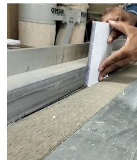
Figure 8: Making tongue by trimming side panels and groove by trimming middle panel
