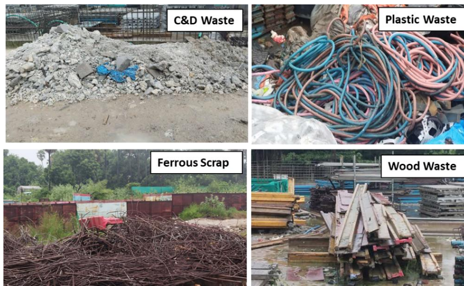
Figure 2: Waste segregation at project sites
