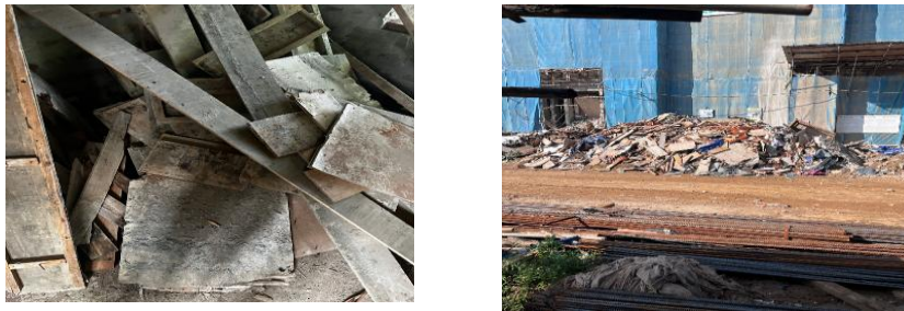
Figure 6: Disposal practices of plywood formwork at the end-of-life in the construction site
