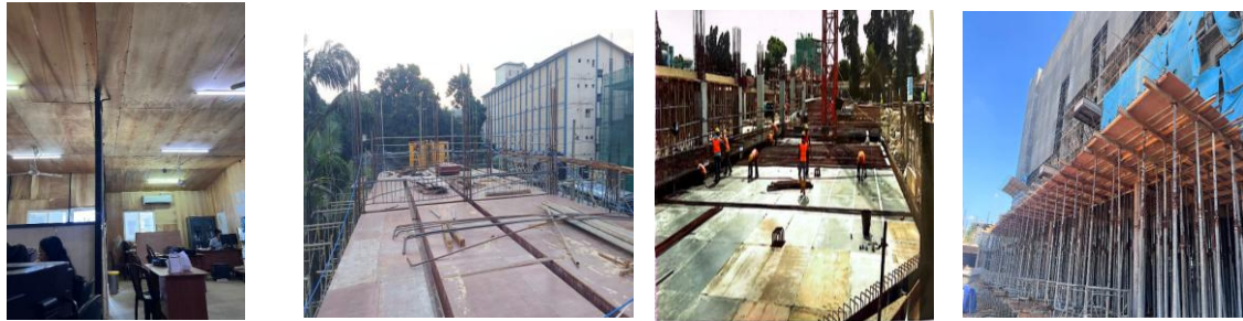
Figure 1 : Typical use of plywood in large-scale construction projects
