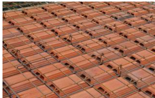
Figure 1: Image showing construction of a filler slab. Source: (Sathya Consultants, 2011)
