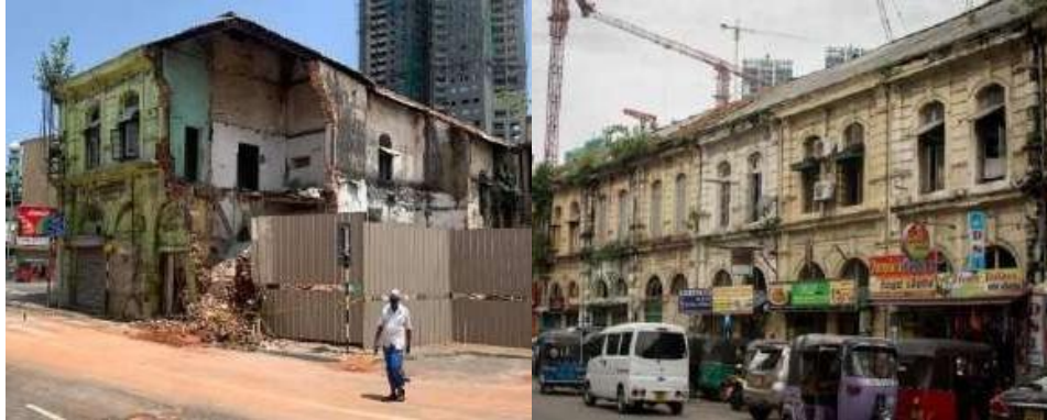
Figure 2 & 3: Demolished state of the De Soysa building.
